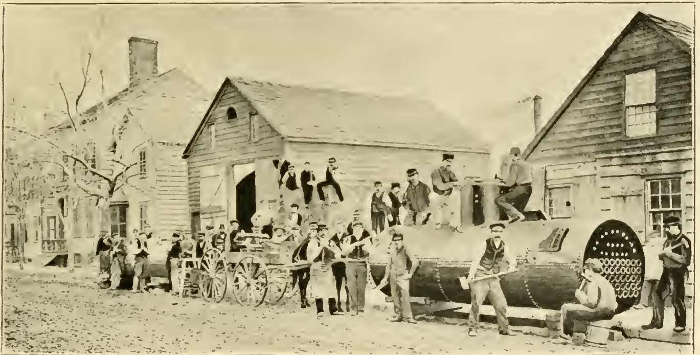
PLANT OF L. J. LYONS & CO., COMMERCE AND CANAL STREETS.
